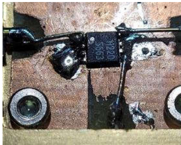
Figure 7 - Closeup of Wiring
